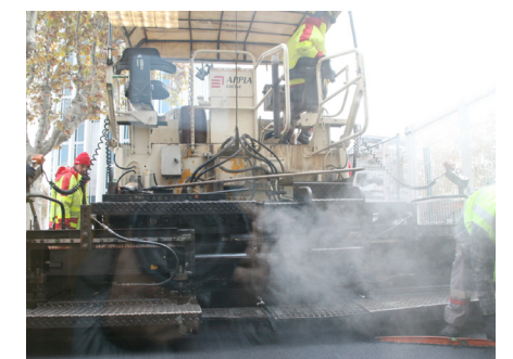
Fig. 2.13.3 Asphalt road-workers are exposed to polycyclic aromatic hydro-carbons
